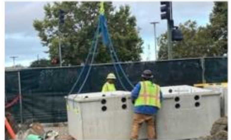
Electric Vault Installation
